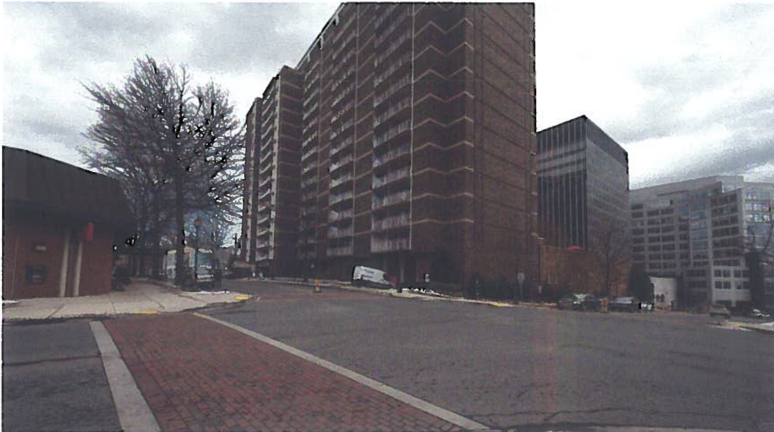
Photo No. 3 above: 15 story Highland House Apartment house occupying an entire block of S. Park Ave. The proposed new building will occupy the entire block of the opposite side of the street.
